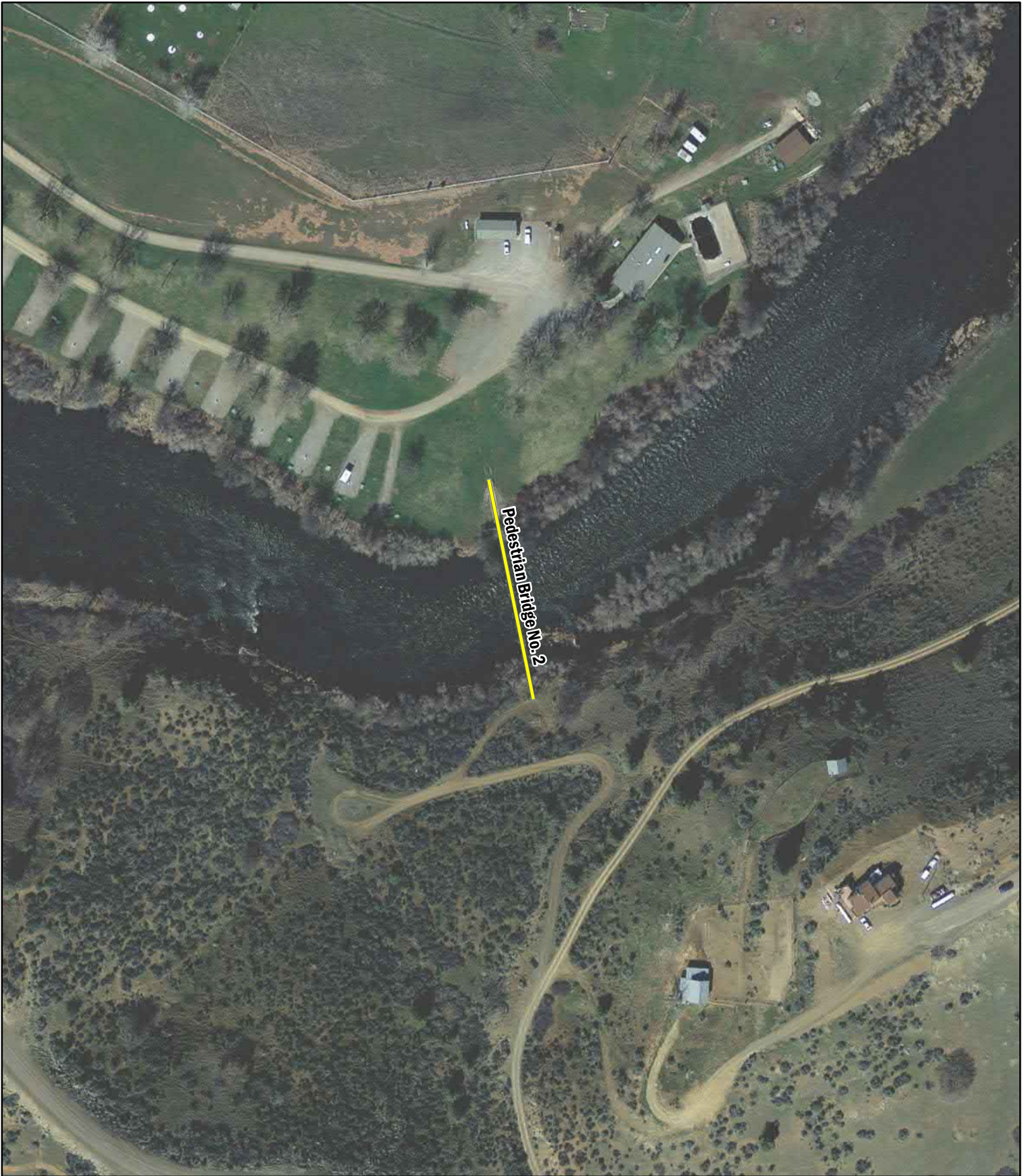
Pedestrian Bridge No. 2
