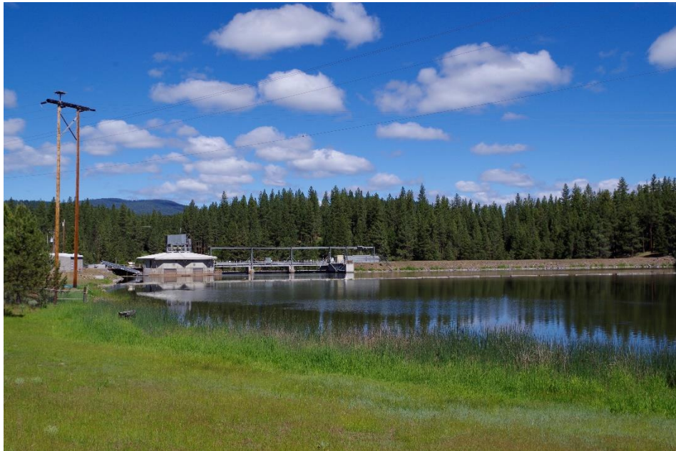
Photograph 7. J.C. Boyle Dam; facing northwest/downstream, 2018.
