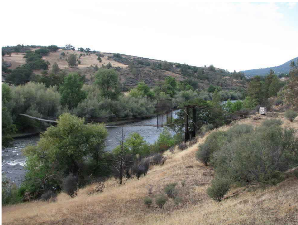
Photograph 1. Pedestrian Bridge 1; view facing south, 2019.
