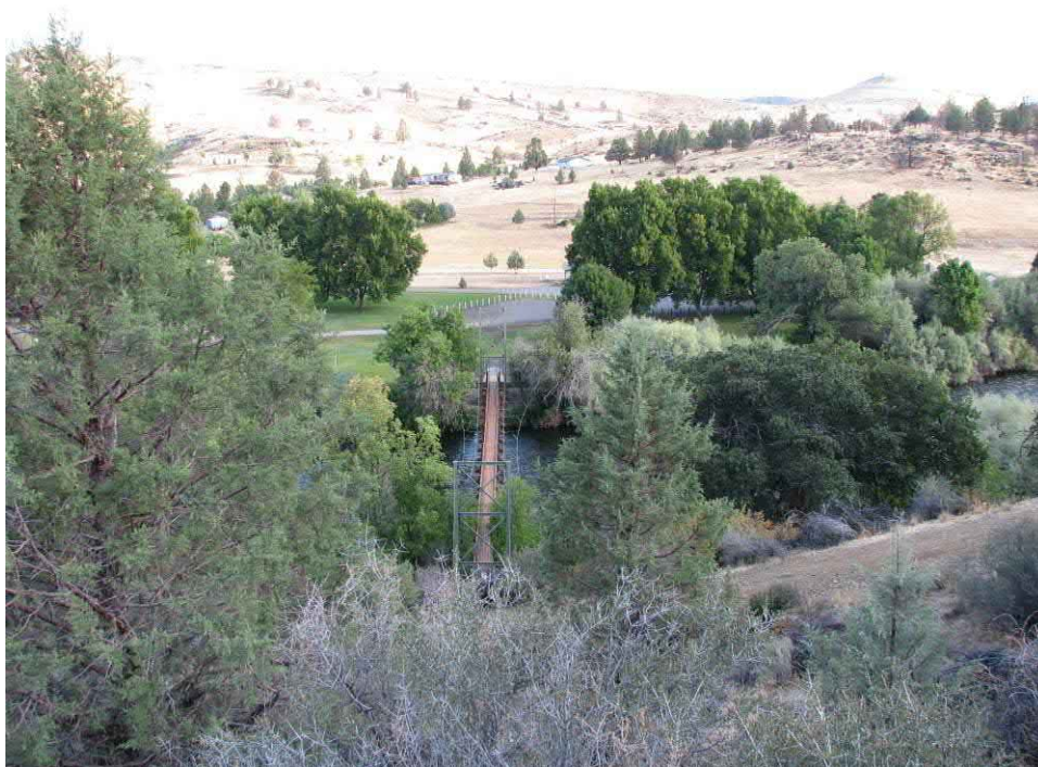
Photograph 1. Pedestrian Bridge 2; view facing north, 2019.
