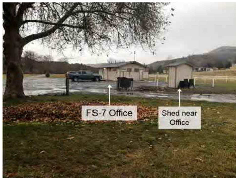
Photograph 2. Klamath River Country Estates Campground office (FS-7), 2019.
