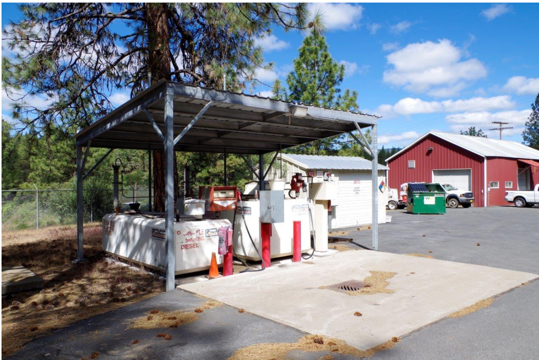
Photograph 4. Fuel Station; facing northwest, 2018.
