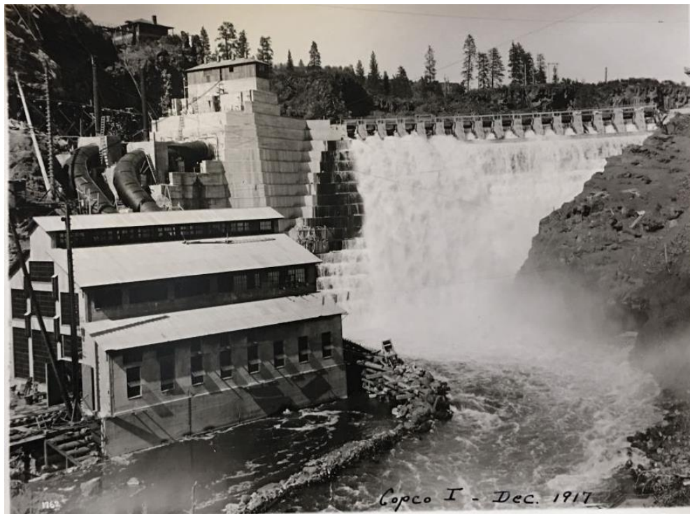
Photograph 2. Copco No. 1, December 1917; facing northeast/upstream (SOHS 1917).
