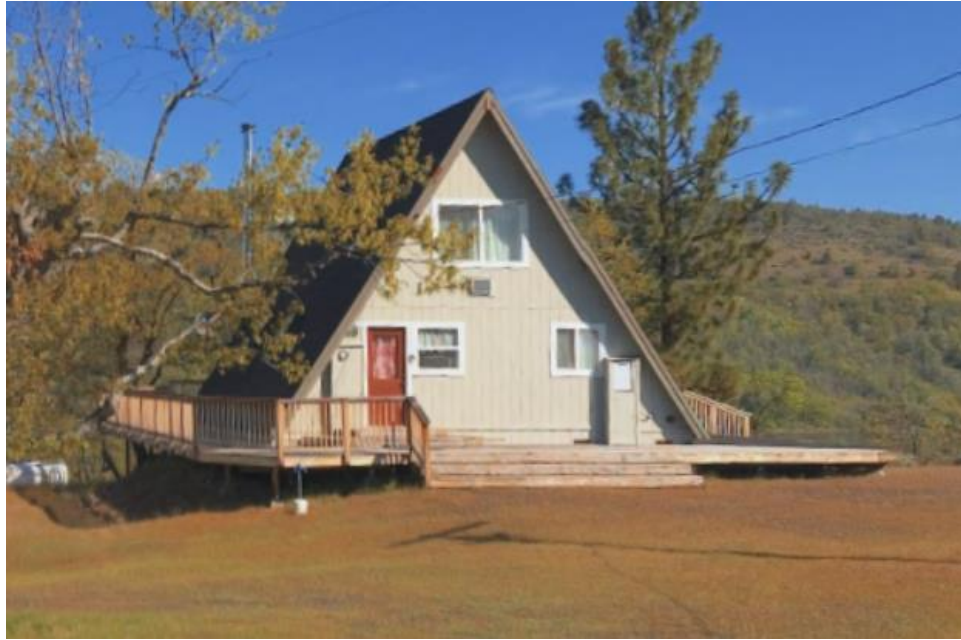
Photograph 3. A-frame cabin at 15830 Patricia Avenue, viewing north.
