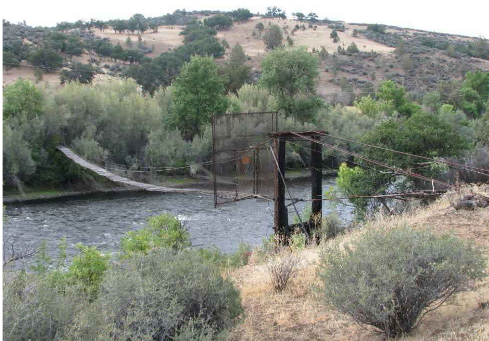
Photograph 2. Pedestrian Bridge 1; view facing south, 2019.
