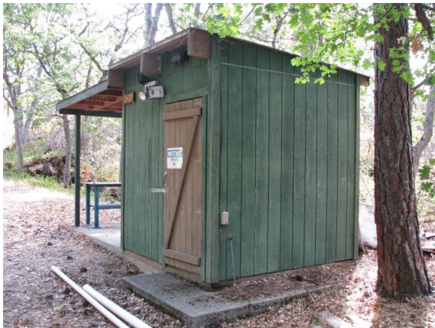
Photograph 5. Shop; view facing south, 2019
