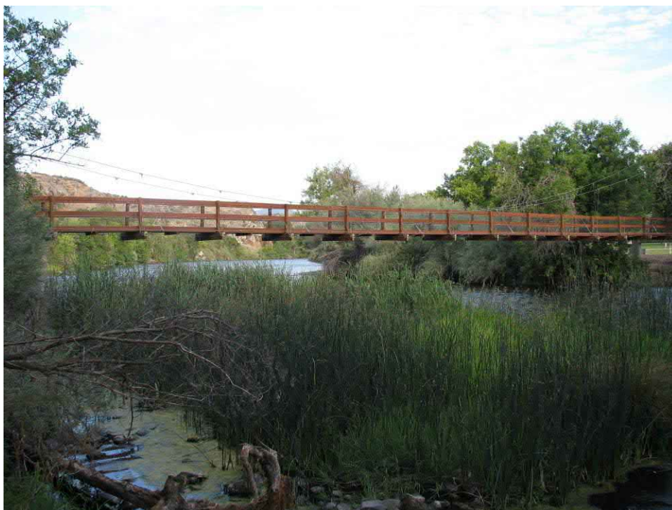
Photograph 5. Pedestrian Bridge 2; view facing west, 2019.
