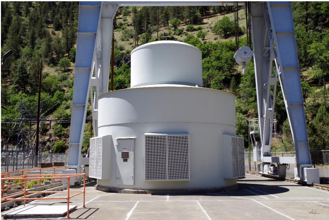
Photograph 4. Powerhouse; facing northwest, 2018.
