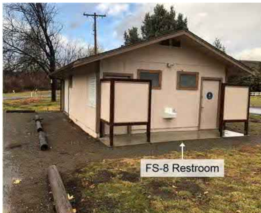
Photograph 3. Klamath River Country Estates Campground restroom (FS-8), 2019.
