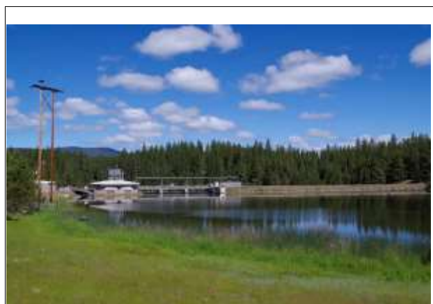
JC Boyle Dam, facing W
